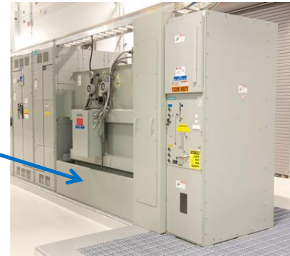
Examples of fluid containment
