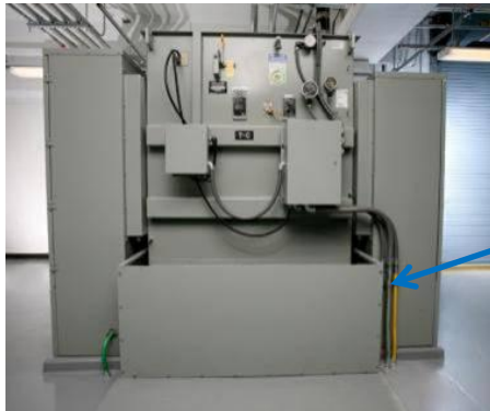
Examples of fluid containment
